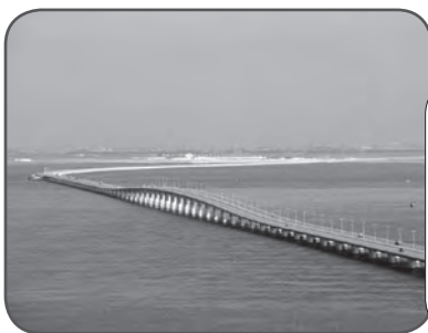
King Fahd Causeway: opened 1986 / actually a series of bridges and dam / 2500 metres long
